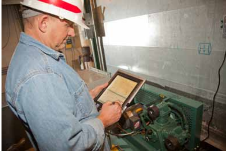
BUILDER uses structured observations designed to evaluate some aspect of performance loss stemming from different mechanisms (distresses), each of which can be measured separately by severity and density. Photo by Louis Bartels
